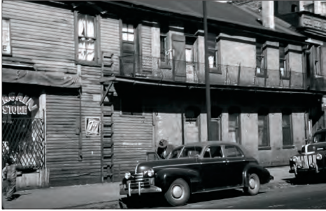
900 West Maxwell Street in 1949: This is now a sports field of the University of Illinois at Chicago (Google Images).
